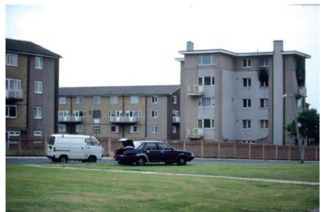
Figure 3: Typical 1950's Dwellings on the estates (Source: Royds Housing Association, 2001)
